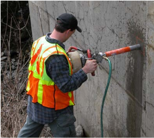
Figure 2 Coring vertical surface. Figure 3 Coring horizontal surface.
