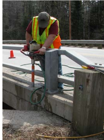
Figure 2 Coring vertical surface. Figure 3 Coring horizontal surface.
