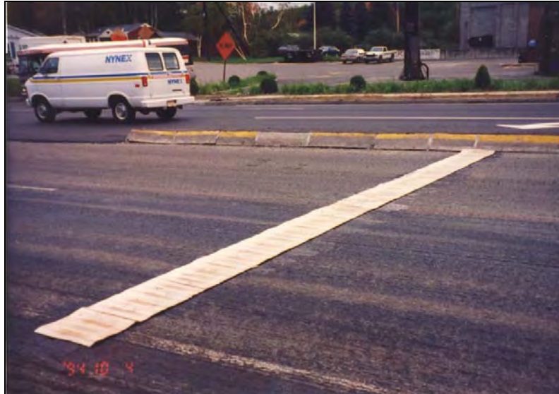
Figure 8 – Hartford PavePrep Installation
