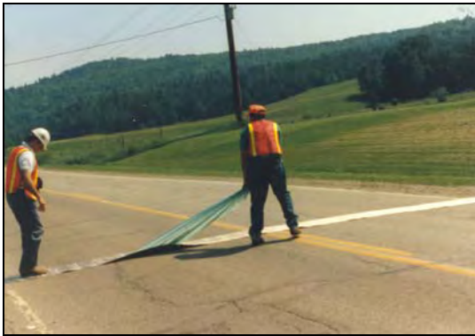
Figure 6 – Lowell MM 6.13 Installation
