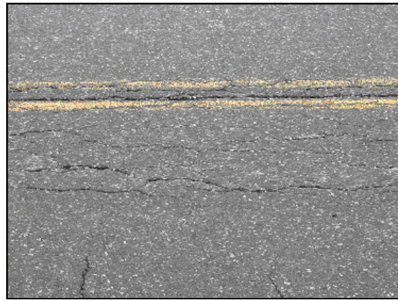
Figure 8 – Eastbound Lane cracking, 2007
