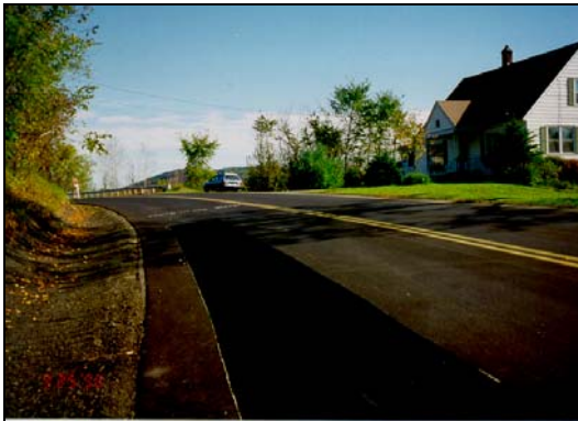
Figure 5 - GlasGrid Placement in Barnet
