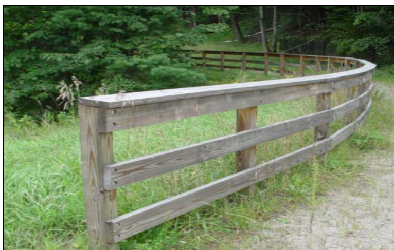
Figure 16: Wood Safety Railing
