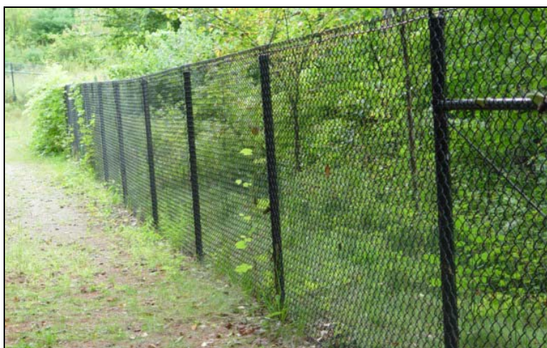
Figure 19: Vinyl Coated Chain Link Fence
