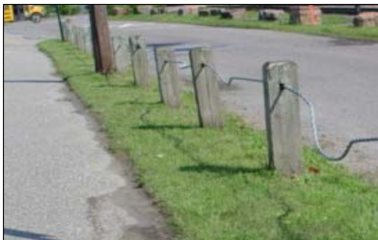
Figure 14: Wood-Cable Fence
