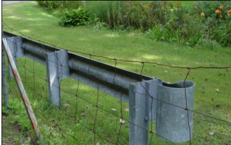
Figure 24: Metal Guardrail
