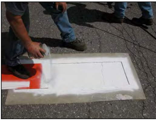
Figure 4 – Application of Glass Beads
