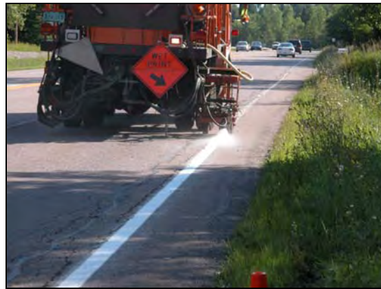
Figure 1 – Application of the White Edge Line
