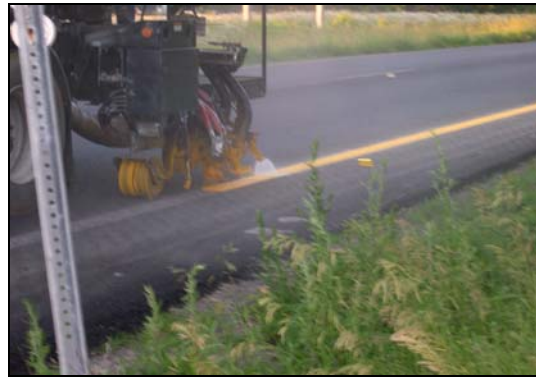
Figure 3- Yellow Edge Line Application
