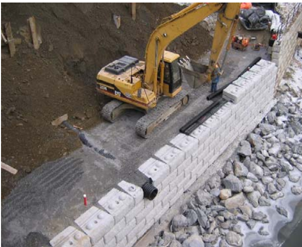
Figure 7: Drainage pipe installed through Redi-Rock™ wall.
