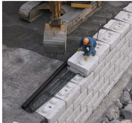
Figure 6: Geogrid installation
