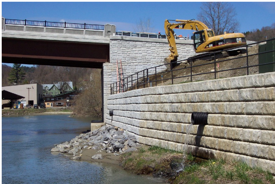
Figure 9b: Completed Redi-Rock Retaining Wall
