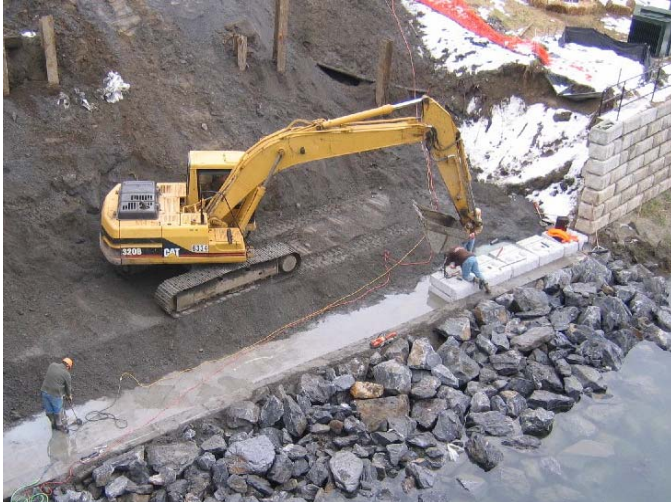
Figure 5: Installation of 1 st row of blocks
