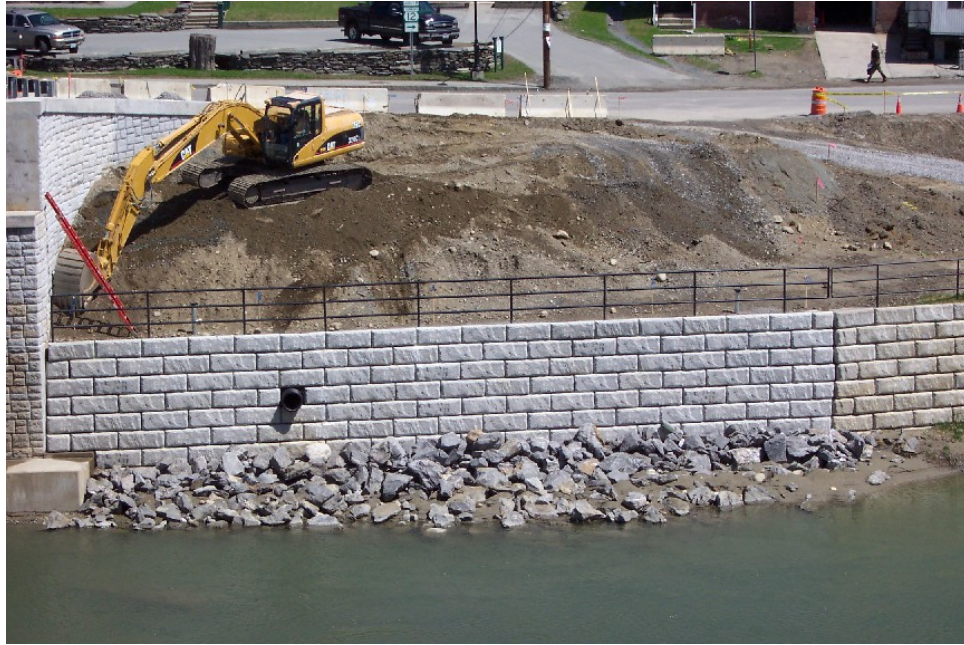
Figure 9a: Completed Redi-Rock Retaining Wall
