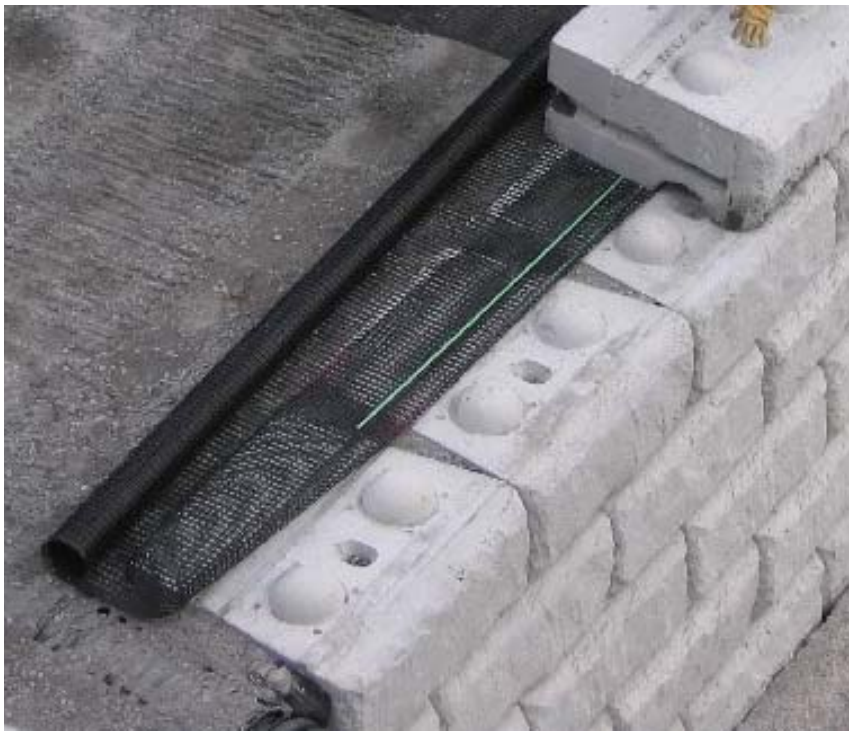
Figure 1: Segmental piece of Redi-Rock wall illustrating the interlocking nodules cast into the blocks and geogrid reinforcement to be embedded in to the soil.
