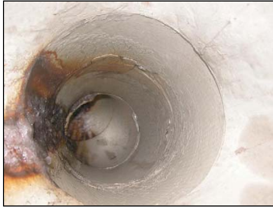
Figure 5 – Iron-Oxide Discoloration
