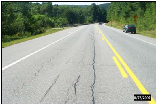
Figure 1 – Test Site 5.9 (Cold Plane)
