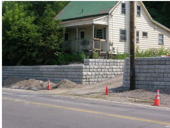
Figure 5: Retaining Walls 1 and 2 constructed with a 90° turn.
