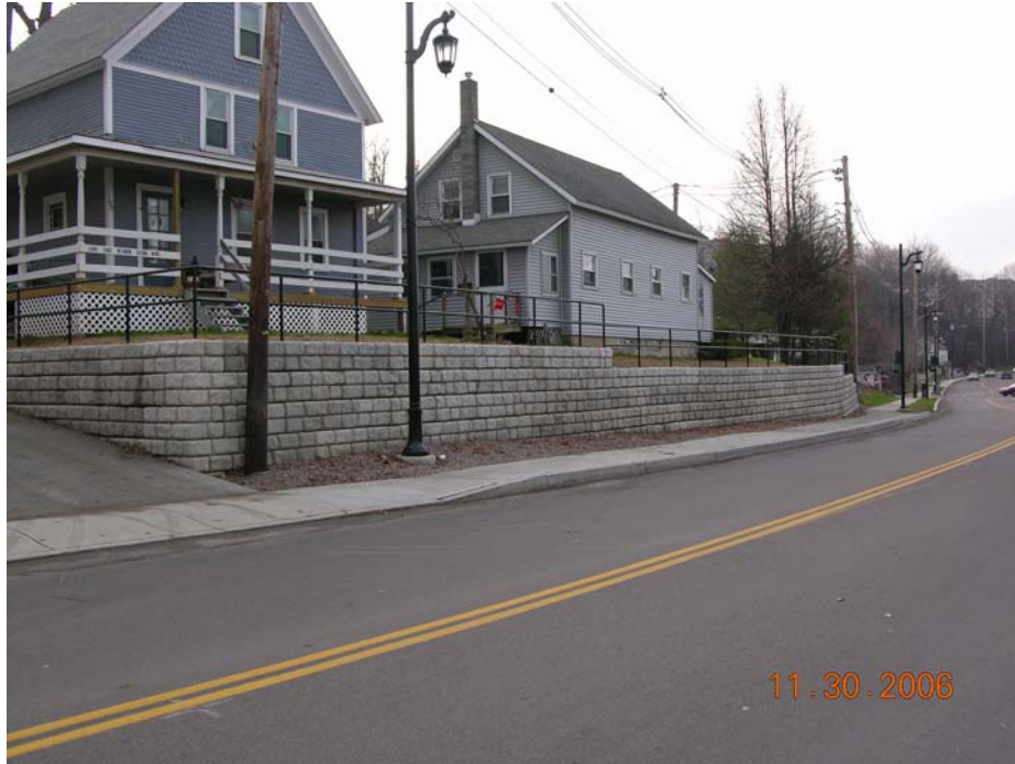
Figure 6: Retaining Wall 1 extended west to include adjacent property.
