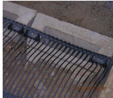
Figure 5: Clips installed through geogrid into modular block.
