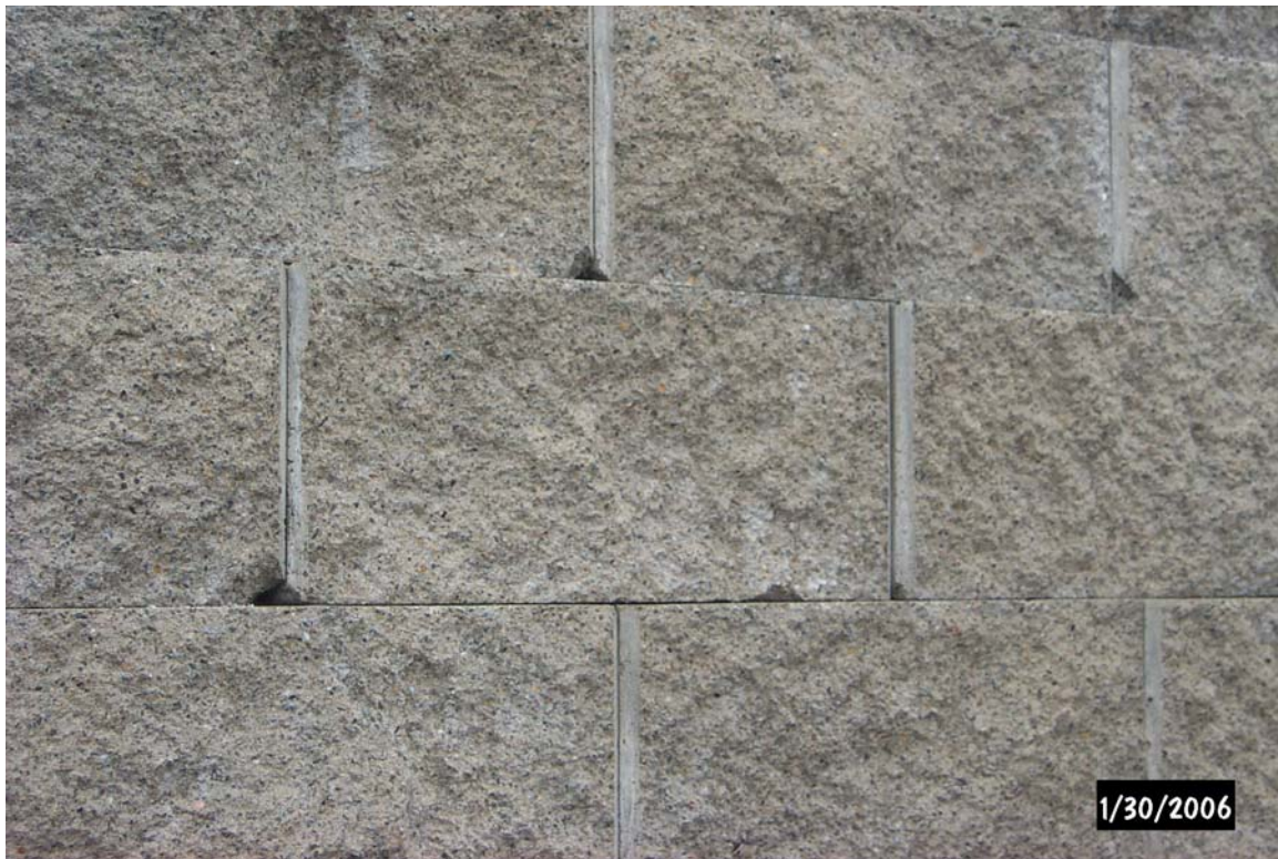
Figure 9 – Blocks with chipped corners
