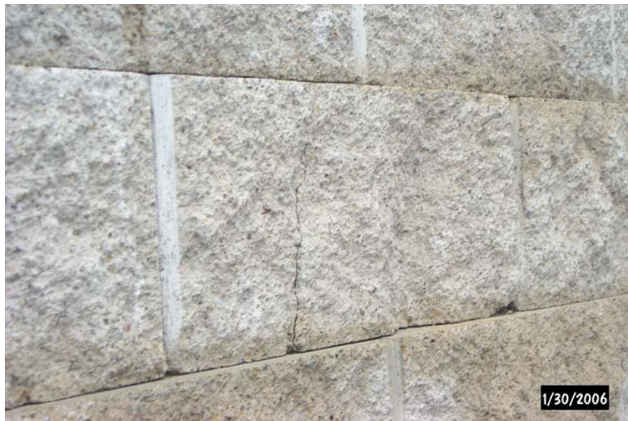
Figure 8b – Vertical fracture
