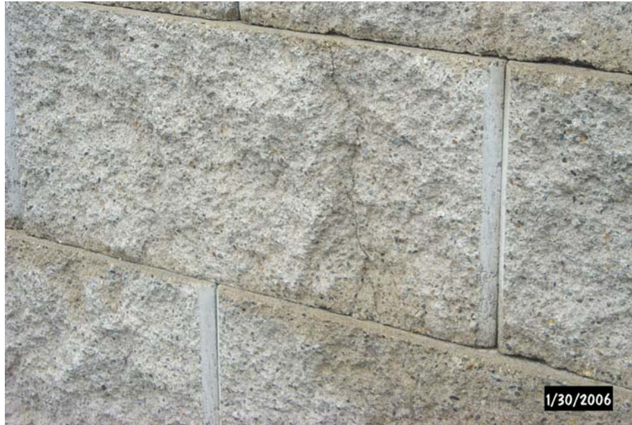
Figure 8a – Vertical fracture
