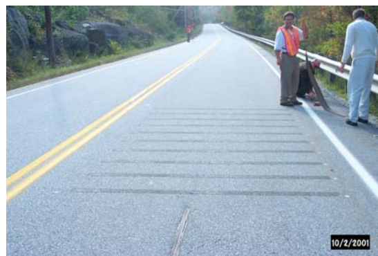
Figure 10. After the rumble strips removal.
