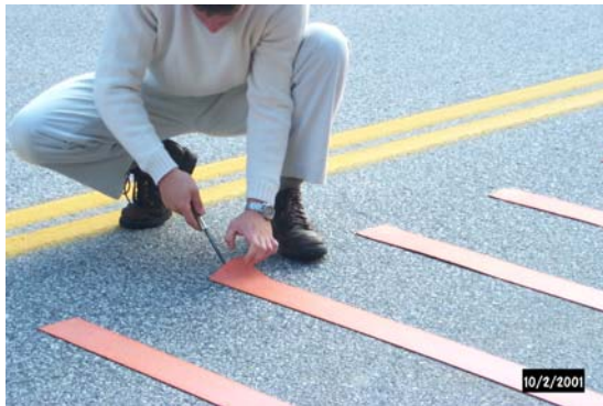
Figure 8. Prying-up the material.
