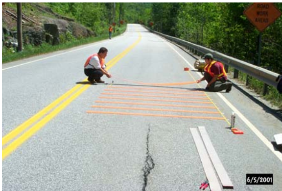
Figure 2. Placing the rumble strips.
