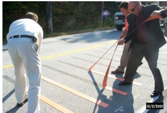
Figure 9. Removing the rumble strips.
