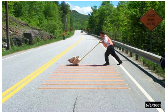
Figure 3. Tamping the rumble strips.
