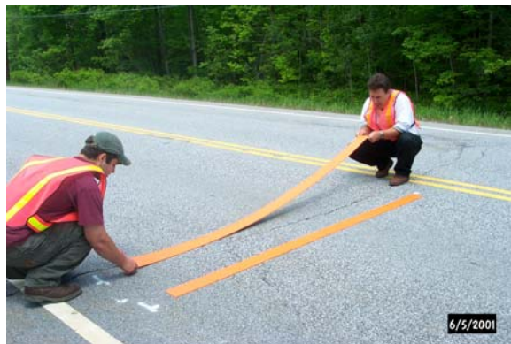
Figure 4. Placing strip over minor crack at most southern test group.
