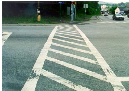
Figure 8. VT Route 12 (Northfield St) – 1998.
