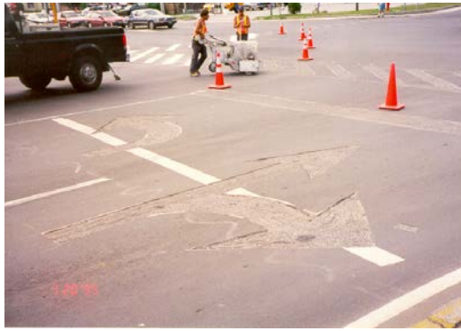
Figure 3. Ground out bituminous pavement.
