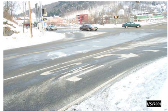
Figure 12. VT Route 12 (Northfield St) – 2001.
