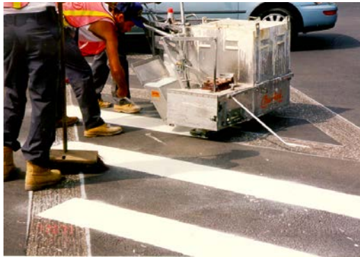
Figure 4. Inlaying thermoplastic material in grooved areas.
