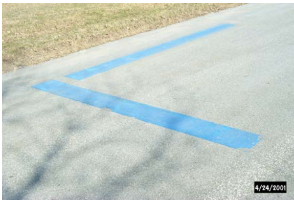
Figure 11. Test Strip A and C after eight months.
