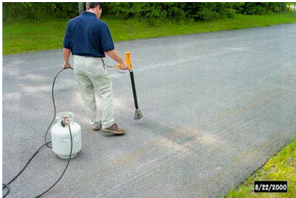
Figure 2. Preheating pavement surface.
