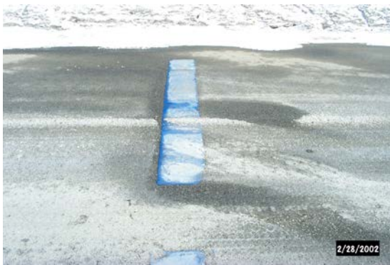
Figure 6. Markings prior to cleaning.
