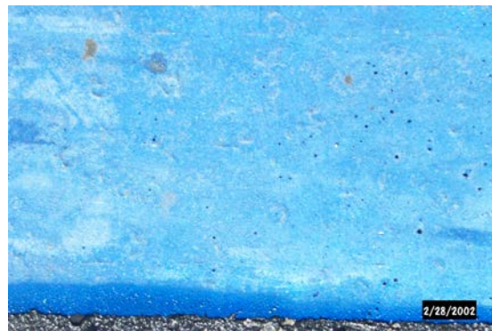
Figure 7. Markings after swept, washed, and dried.
