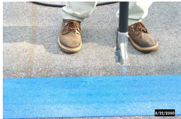
Figure 3. Heating preformed thermoplastic material.
