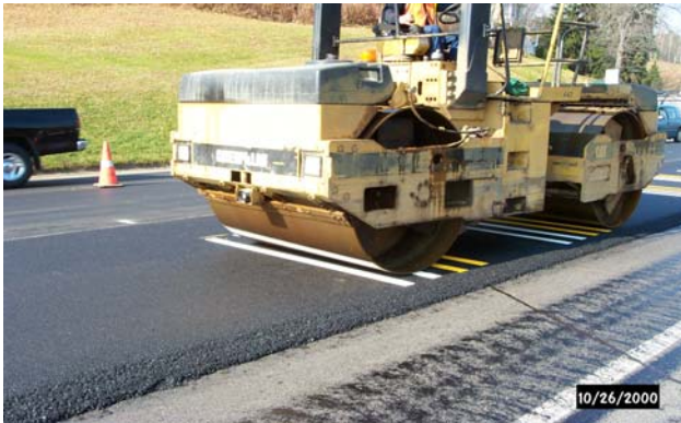
Figure 4. Compacting tape with roller. (Photo taken October, 2000)
