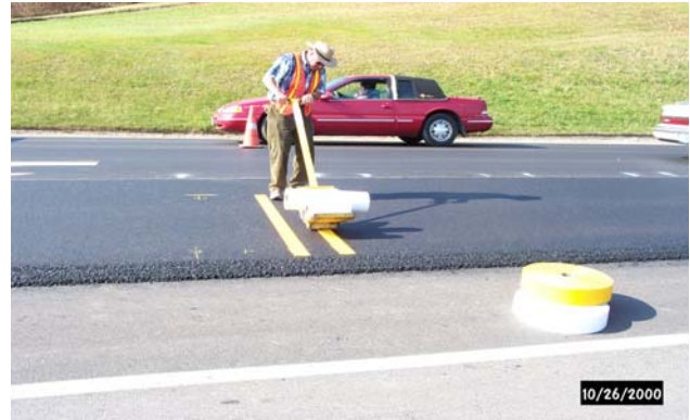
Figure 3. Securing tape with hand tamper. (Photo taken October, 2000)
