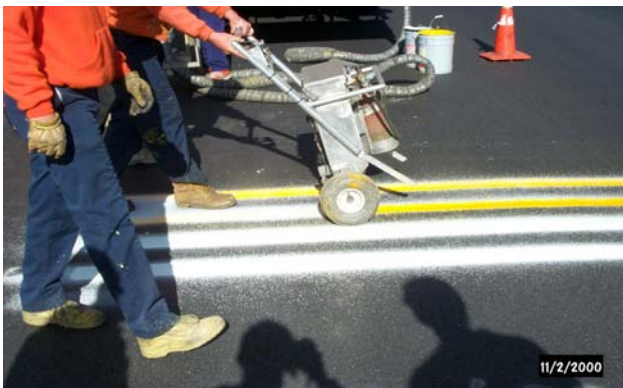
Figure5b. Application of glass beads to epoxy pavement markings. (Photo taken November, 2000)
