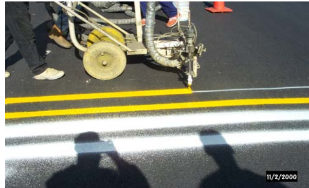
Figure 5a. Application of epoxy pavement markings. (Photo taken November, 2000)
