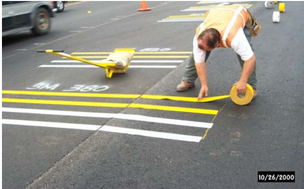
Figure 2. Placement of permanent tape. (Photo taken October, 2000)
