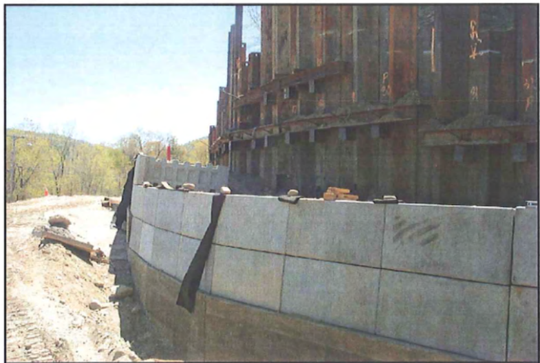
Figure 3. STA 0+320 Fill Wall Constructed in a Cut Slope Retained by Sheet Piling
