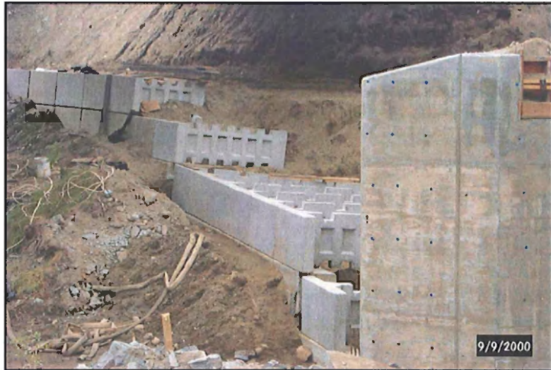
Figure 4. STA 0+800 Fill Application Next to Bridge Abutment
