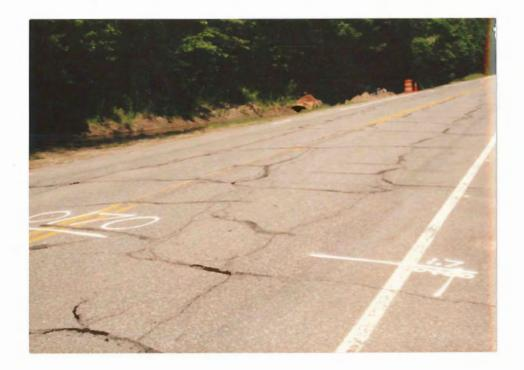
Severe low temperature thermal stress cracking on VT Route 18 in Waterford
