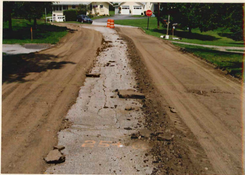
STATION 25+00 BEFORE THIRD PASS OF RECLAIMER
