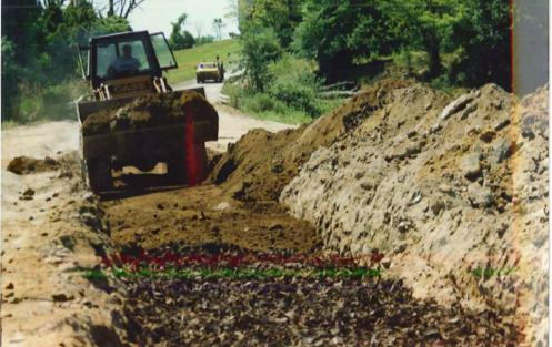
Leveling the tire chips with a backhoe to obtain a 9" to 12" layer.
