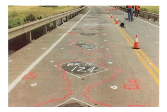
Condition of NB lane on August 24, 1989. Red lines indicate the perimeter of concrete delaminations. White rectangles outline areas to be saw cut and patched.
