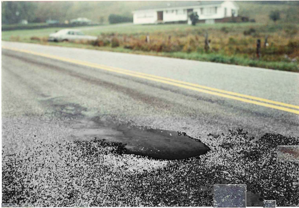
This photo shows a patch which has been applied to correct shoving in the recycled pavement overlay.
