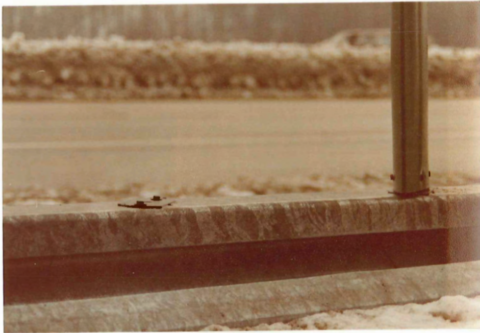
Vertical portion of bracket broken off
