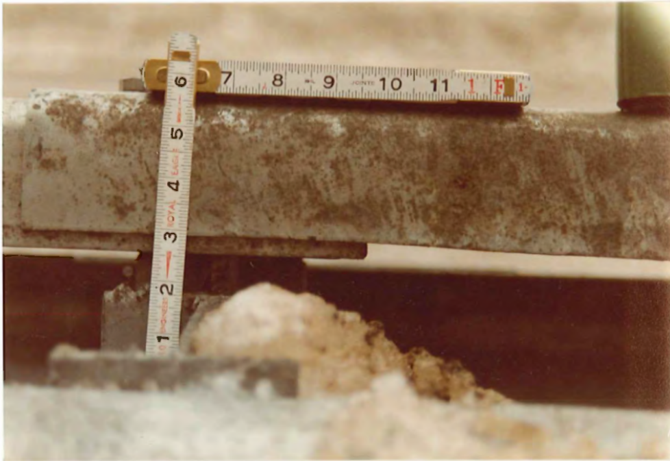
Tilted mounting plate bracket.
