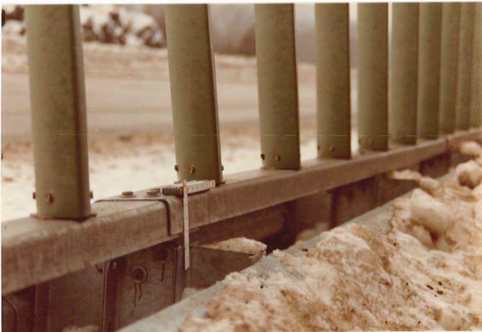
Tilted mounting plate bracket.
