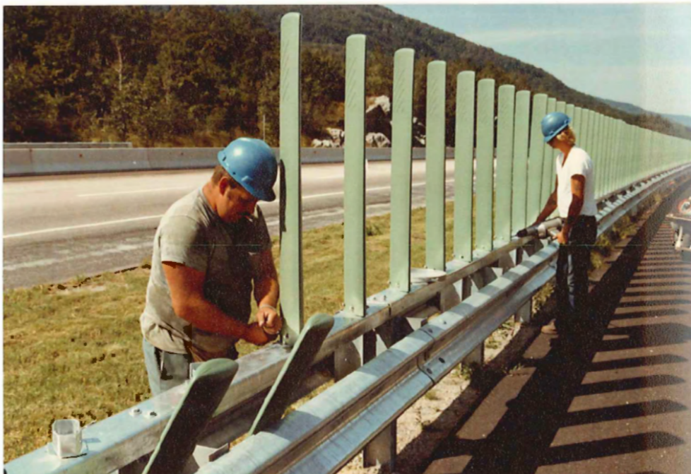
Installing Glarefoils
