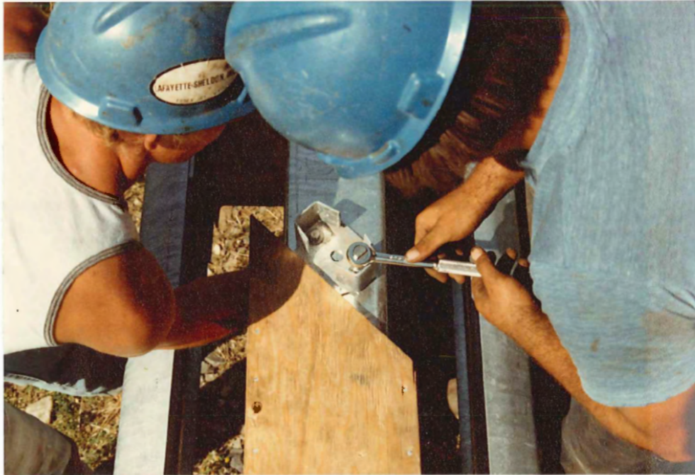
Installing Glarefoil Brackets
