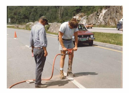
The hole was blown clean with compressed air and then moistened using a pail of water and a six inch brush. SET-45 patching material was used to hold the markers in place. A small amount of material was placed into the hole and the marker was dipped into the bucket of water then placed in the hole and pressed into place using a template. The template was provided by the manufacturer. The following photographs show examples of installation procedures.
