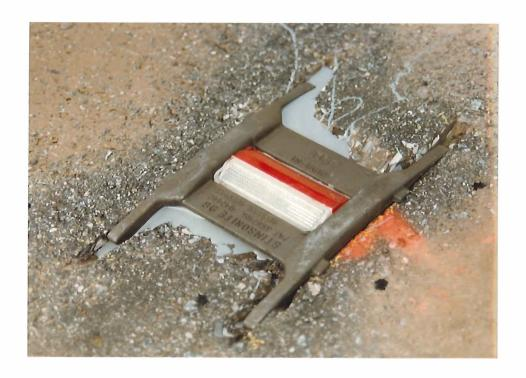
An attempt to remedy the problem by adding epoxy to the high side often caused it to run out onto the pavement. This problem was encountered on many of the markers as shown in the photograph on the following page.
