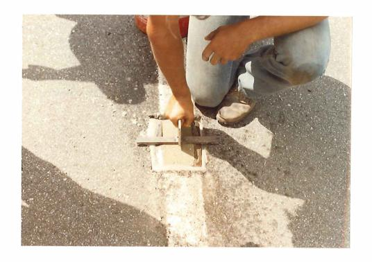
When the marker was pressed into the pavement with the template or leveling tool, the patching material would flow up around the sides of the marker. The excess patching material was then smoothed out or removed using a trowel. Caution was needed to mix the SET-45 properly in order to avoid a mix which was too wet, causing the marker to sink below the pavement surface.
