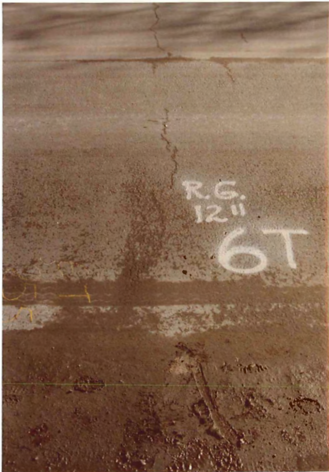
Photo #6 - Roadglas has reflected through but crack is tight and does not run full width of the lane. Crack was treated with 12 inch Roadglas.
