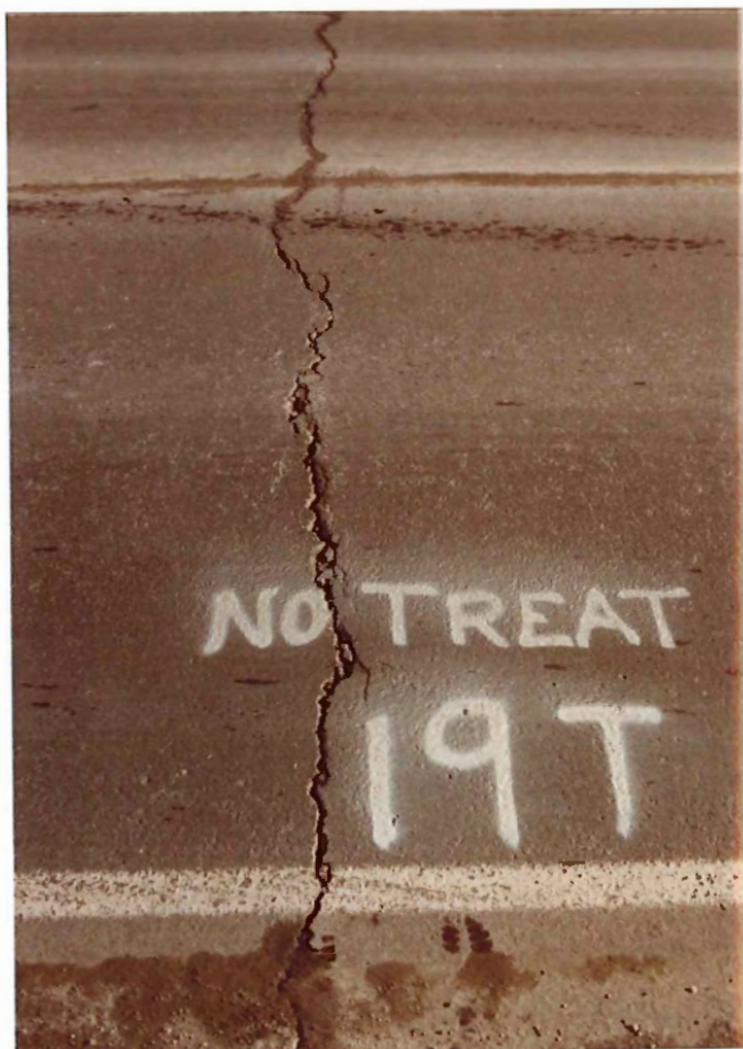
Photo #8 - Example of untreated crack - failure.
