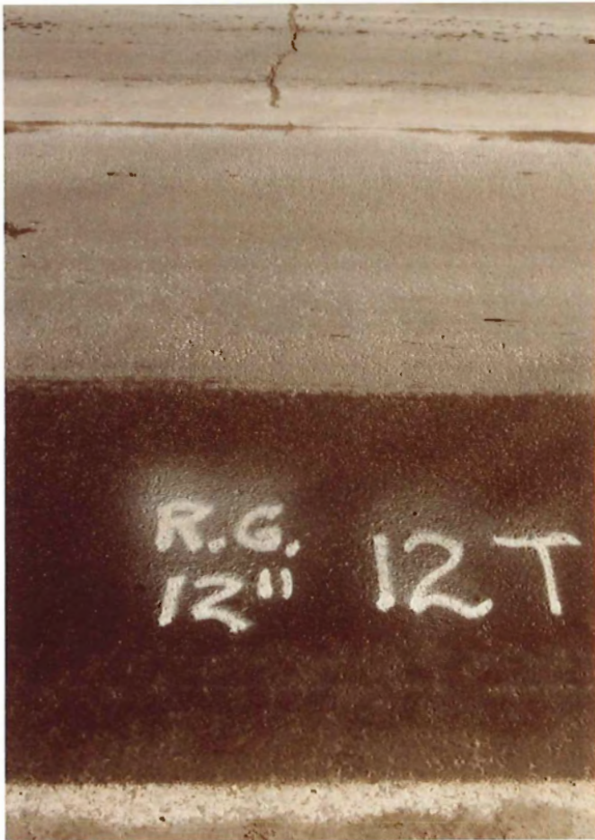
Photo #5 - example of Roadglas performing well. Crack was treated with 12 inch Roadglas.
