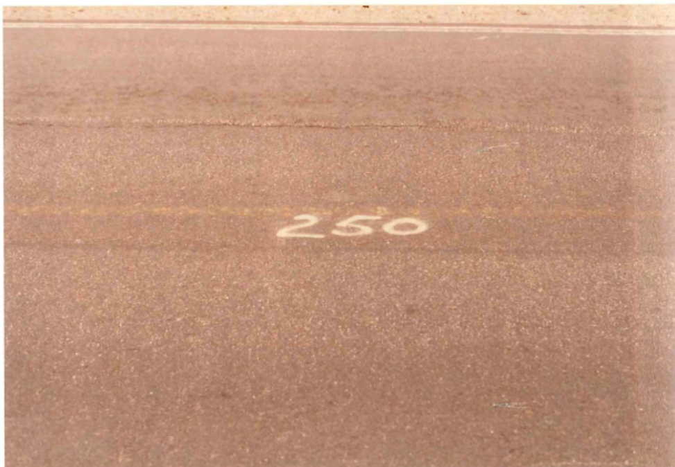
June 1982 Pavement Condition at Station 250 Modified Mix Foreground - Standard Mix Background
