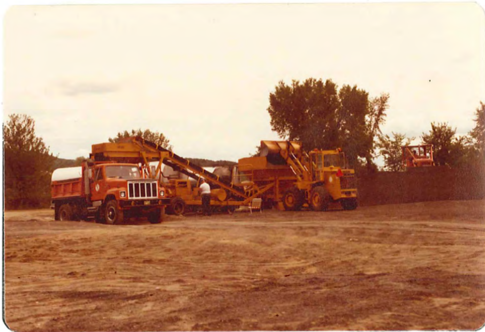
Portable Mixer In Operation
