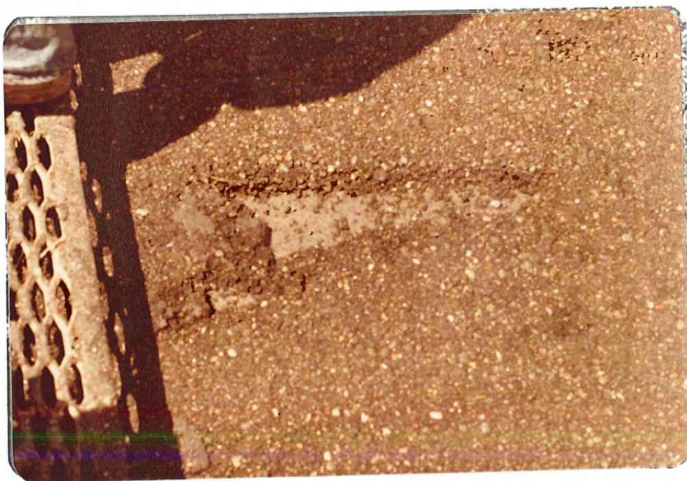
Drag Marks Caused by Build-Up of Material On Screed
