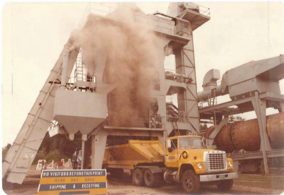
Figure 9 Maximum Emissions At Pug Mill Due To Venting Of Steam
