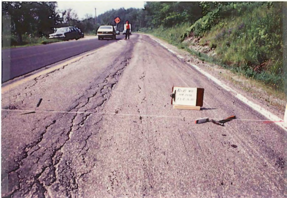
Figure 2 Condition Of Old Pavement Surface On Test Section No. 4
