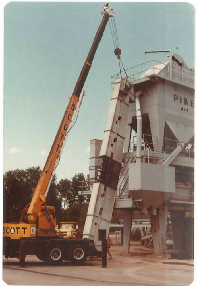
Figure 4 Installation of Elevator
