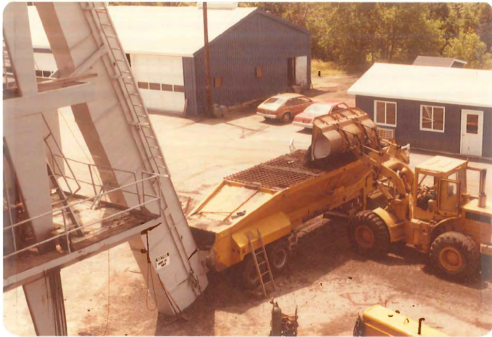
Figure 6 Feeding Reclaimed Material to Weight Hopper
