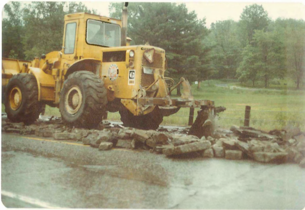
WORKING LARGE CHUNKS TO THE SURFACE
