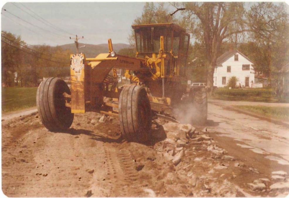
WINDROWING MATERIAL FOR PULVERIZATION
