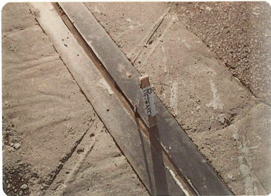
Evazote 50 separated from the steel plate for the full depth of the material.
