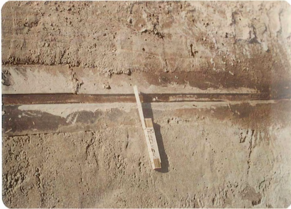
Evazote 50 separated from the steel plates in an alternating pattern.
