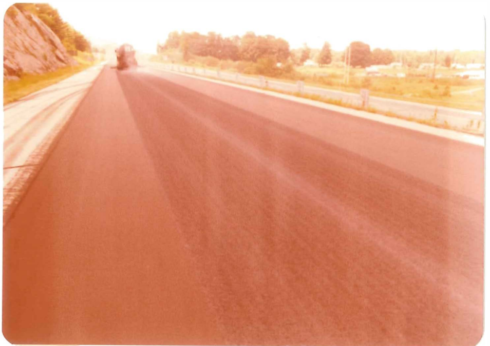
Streaks or ridges in the asphalt rubber application
