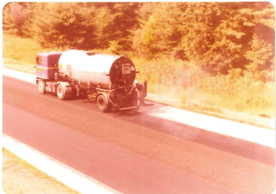
Overlap on Longitudinal Joints
