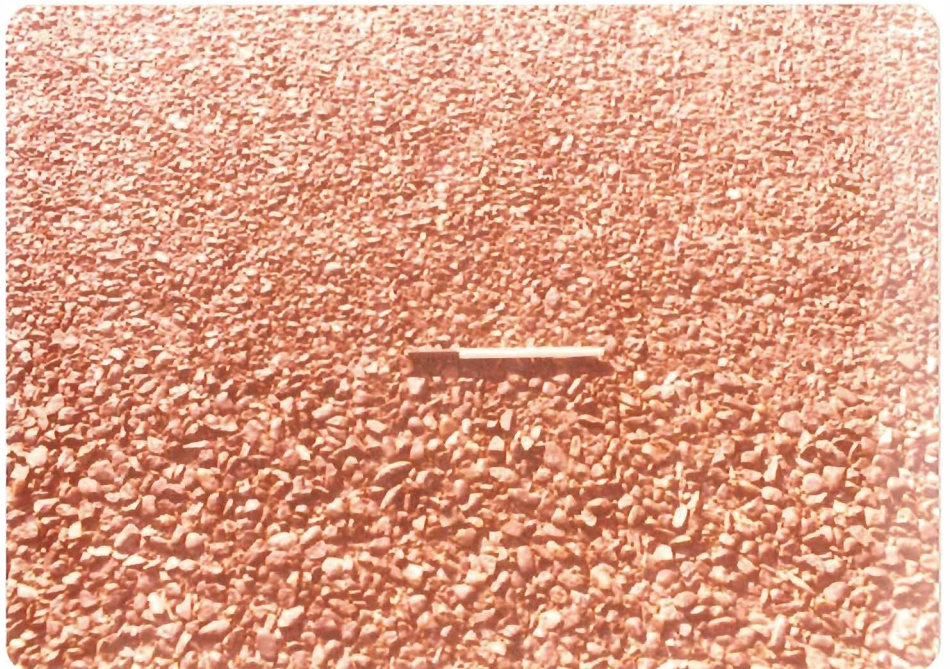
Abutting areas of 3/8 and 1/2 inch cover stone.
