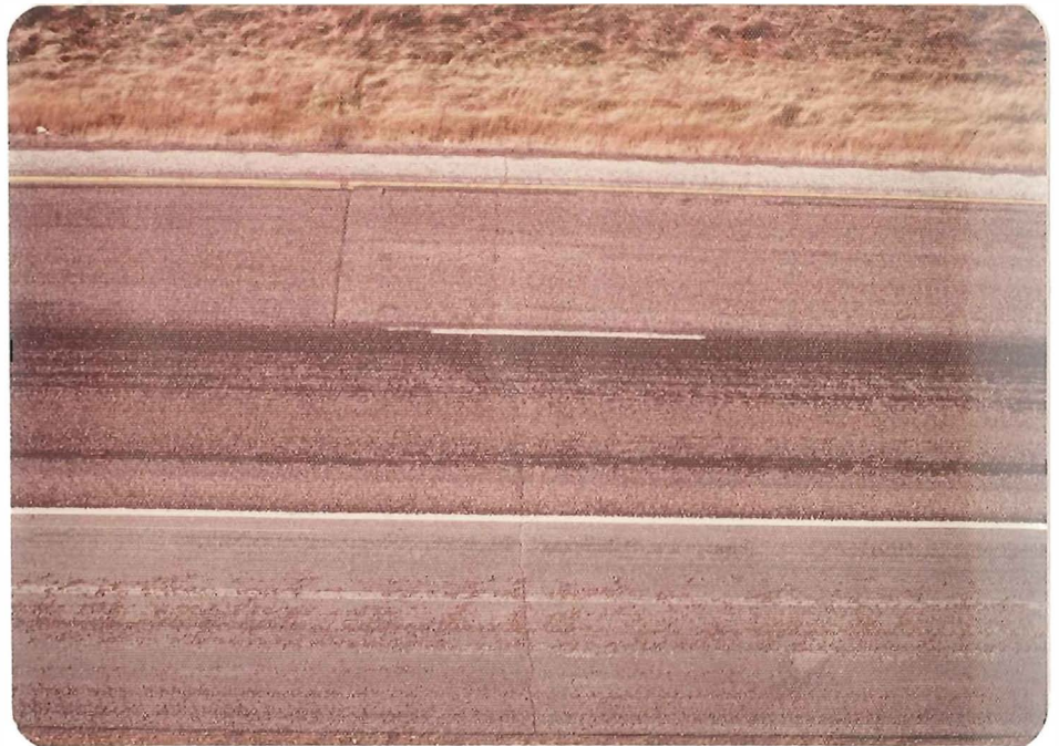
Note loss of cover stone and transverse cracks visible through the surface treatment.
