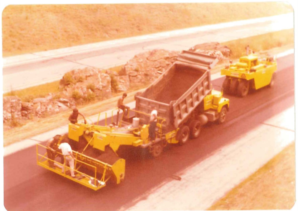
Cover stone application and roller operation
