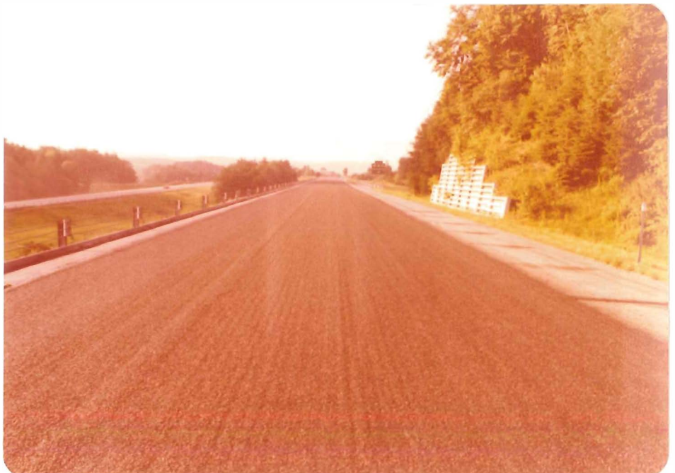
Streaks or ridges in the cover stone
