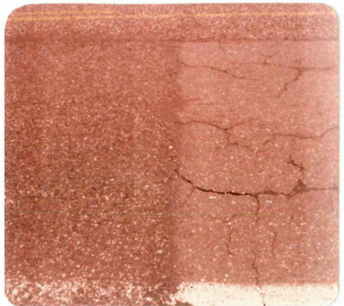
Area Exposed to Traffic For 9 Months, Note Cracks in Abutting Untreated Area
