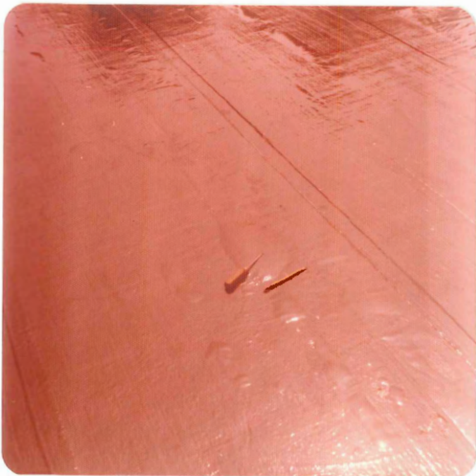
Air blister concentrations resulting from compaction of the No. 10 membrane
