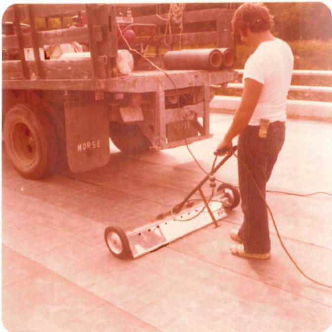
Heating Membrane to create adhesion to concrete
