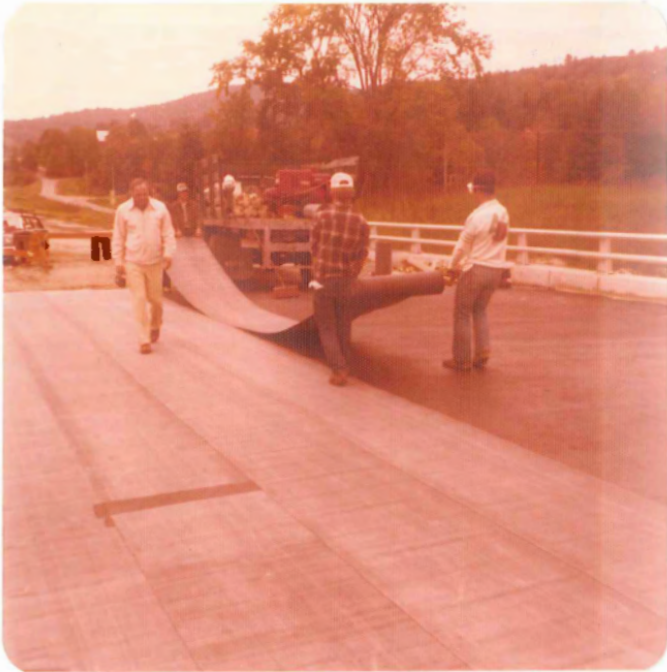
Placing Tri-Ply Membrane
