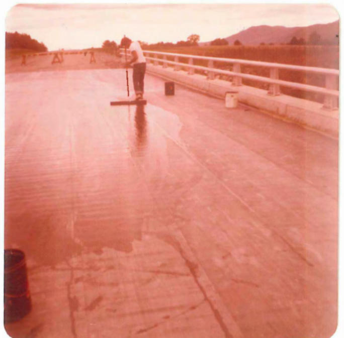
Applying RS-1 emulsion over membrane
