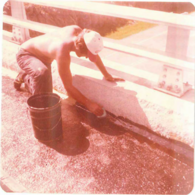
Placing Polyurethane Sealant along curb line
