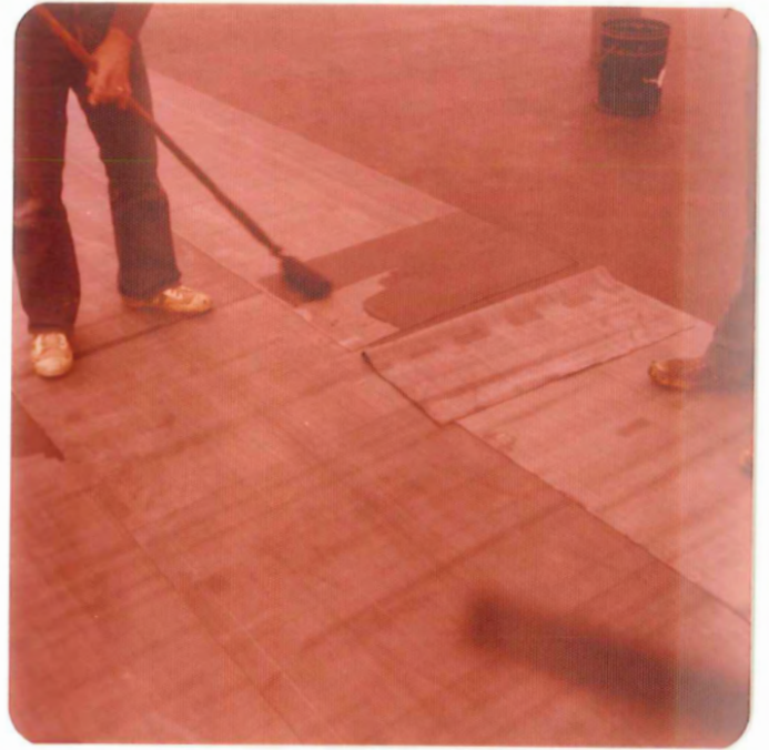
Priming Membrane at end laps
