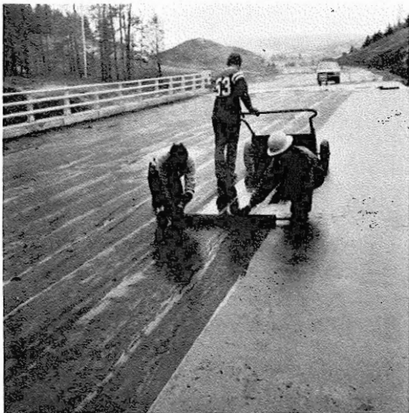
Placing glass fabric in first coat of hot asphalt.
