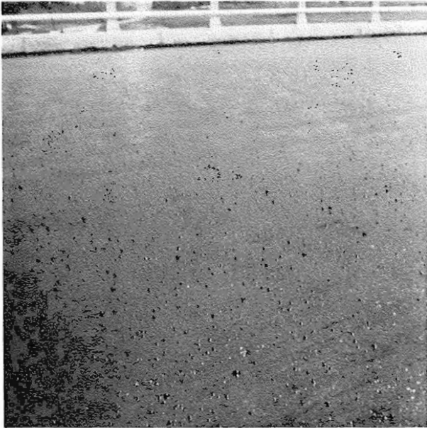
Bubbles up to \frac{3}{4} inch in diameter appeared in the cut-back asphalt prime coat shortly after application.
