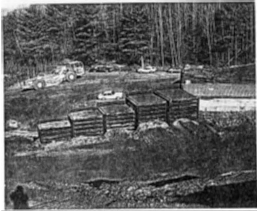
Binwall Backfilled
