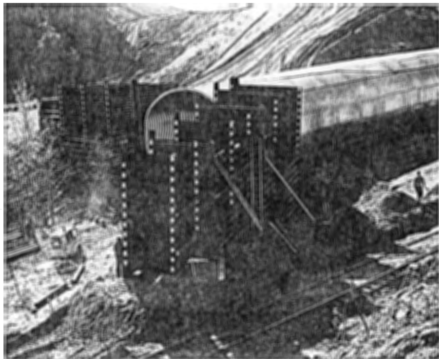
Bin Type Retaining Wall
