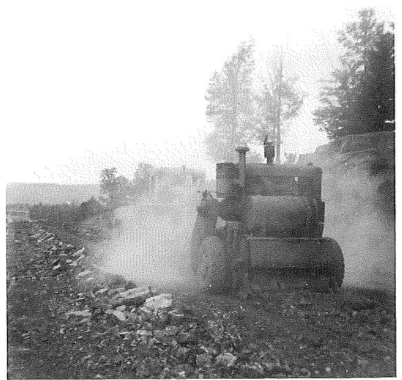
Motorized pulverizer drawn by front-end loader.
