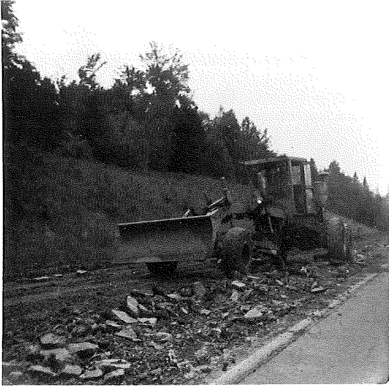
Windrowing pavement between shoulders during pulverization process.
