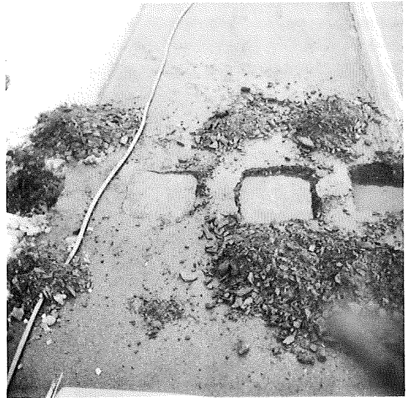
MM 172/95. While opening test pits — free water seeking own level. Note snow on bank. December, 1973.
