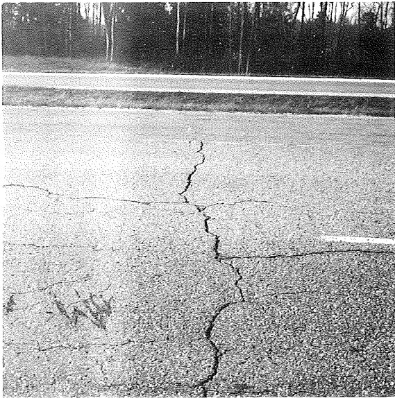
MM 172/95. Condition of pavement in area to be pulverized. October, 1973.
