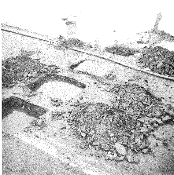
MM 172/95. 2' x 2' holes separated by 1' to edge of shoulder. Running out of third hole. December, 1973.
