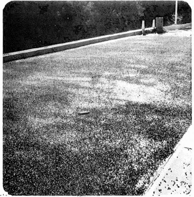
Eastbound lane complete. Note where stone chips penetrated into the Gussasphalt.
