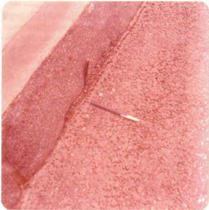
Loss of seal at curb line
