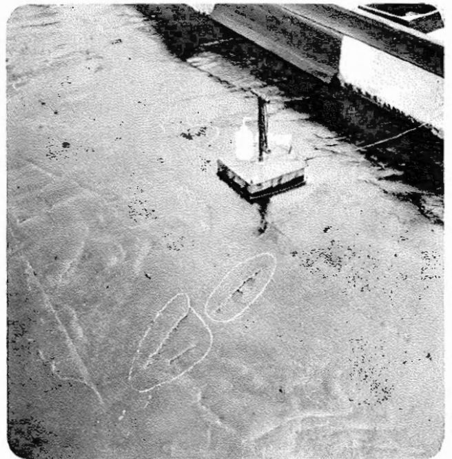
Voids in mastic asphalt prior to touch-up.
