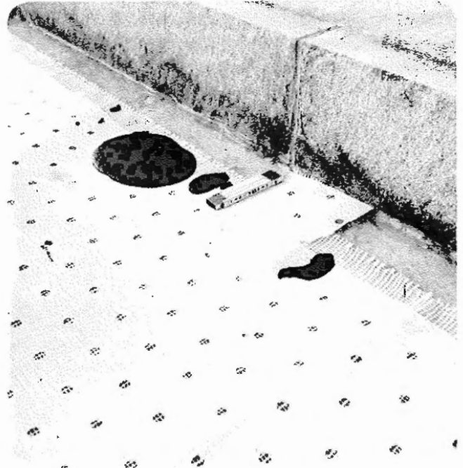
Fiberglass vapor release system. Note extension of system over drain tube near curb face.
