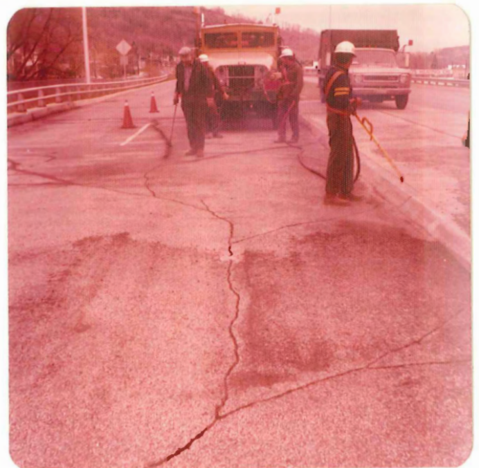
Routing and burning cracks prior to sealing
