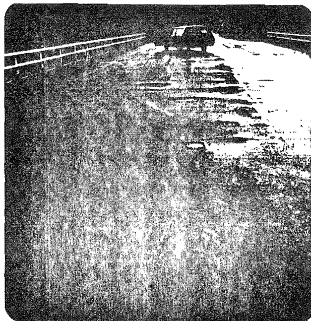
Blisters in Membrane and first course of pavement.
