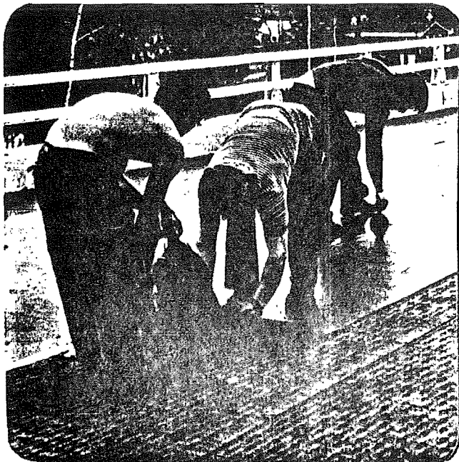
Rolling Hyload Membrane into application of hot roofing grade asphalt.
