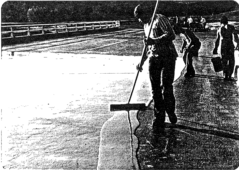
Applying 2-component polyurethane over epoxy prime coat.
