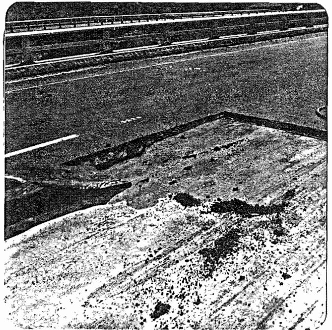
Measurable amounts of water were noted on the concrete in areas where the impervious membrane was not bonded.
