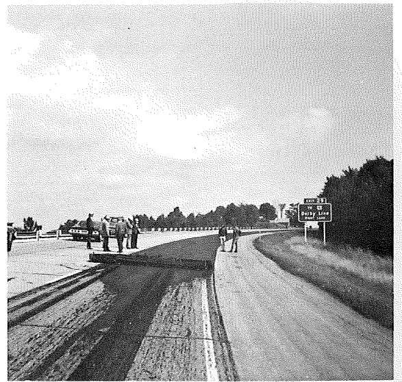
Laying first course of SRI. Note crack filler and shoulder overlap.
