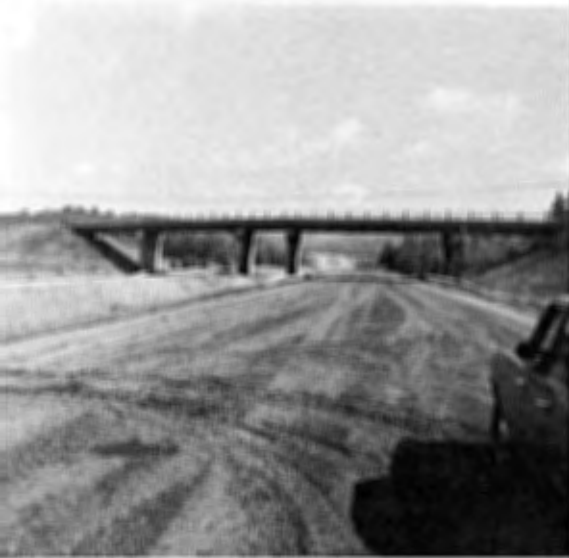
View of pulverized area after grading prior to addition of emulsion and rolling.
