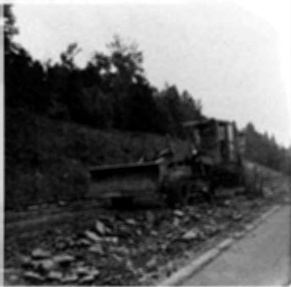
Windrowing pavement between shoulders during pulverization process.
