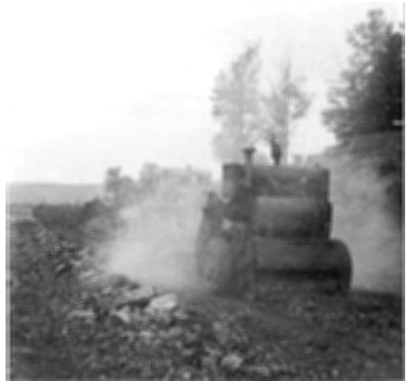
Motorized pulverizer drawn by front-end loader.
