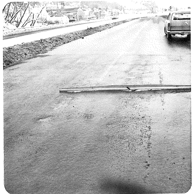
Depressions in the finished surface at locations where the mix was dragged.
