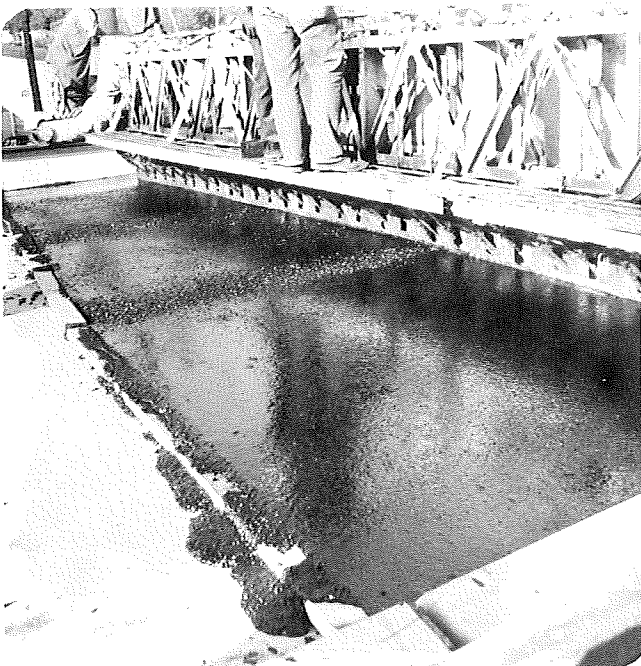
Difficulties with the leveling screed dragging the mix.
