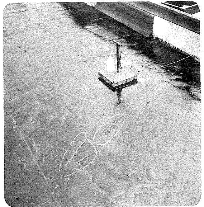
Voids in mastic asphalt prior to touch-up.
