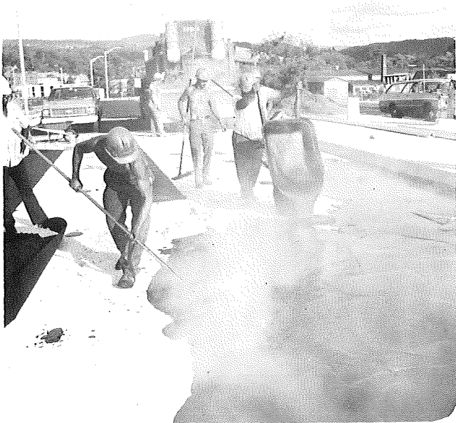
Placing and spreading mastic asphalt with squeegees.
