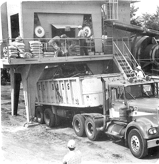
Adding the mineral filler into the pugmill by hand.
