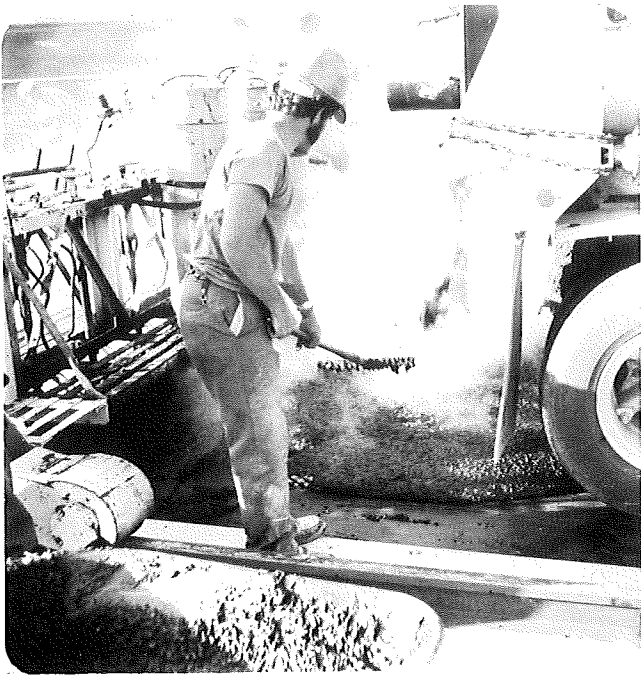
Placing the Gussasphalt directly in front of the leveling screed.
