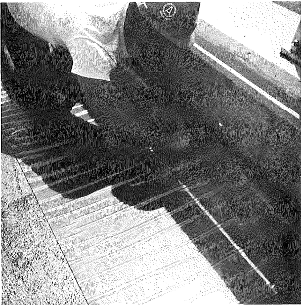
Pressing the membrane into the mastic at the curb line with a one inch diameter wallpaper roller.
