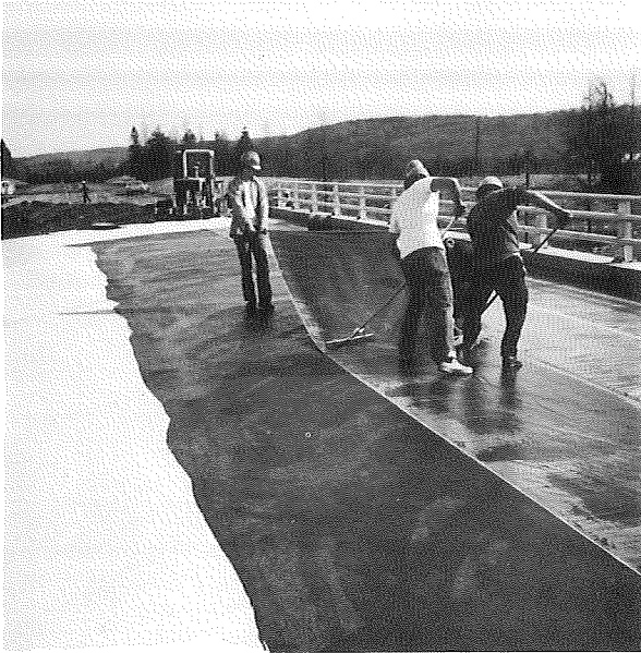
Using squeegees to prevent entrapment of air beneath the membrane during application.
