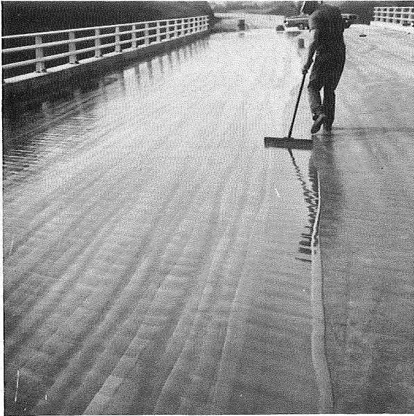
The application of multiple coats of epoxy reduced but did not eliminate all pinholes.
