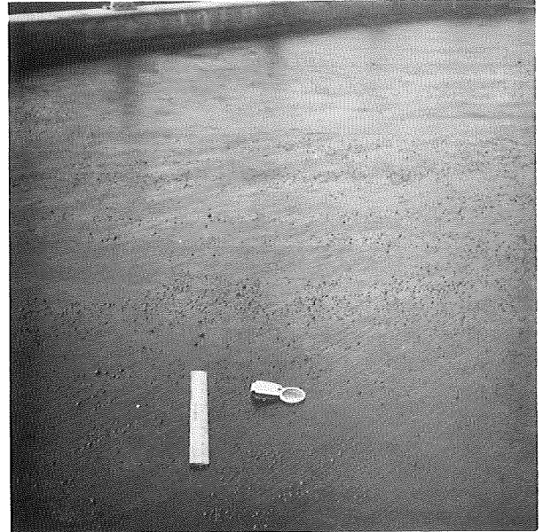
Air bubbles in the solvent cut prime coat were broken with a squeegee prior to placing the membrane sheets.
