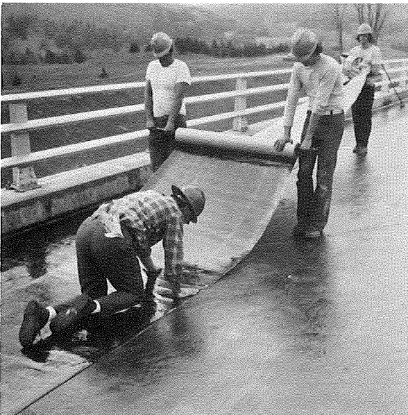
Placing 48 inch wide membrane sheet with 2-1/2 inch edge overlap. Ripples which remained in the membrane did not cause any difficulties with the pavement application.
