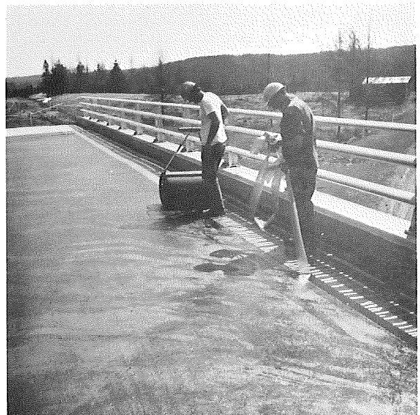
Rolling the membrane and removing the polyethylene film to expose the self sealing edge.
