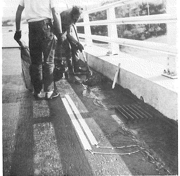
Placing glass fabric in the first coat of asphalt along the curb. Note moisture sensing copper foil strips placed beneath the membrane to detect the passage of moisture.
