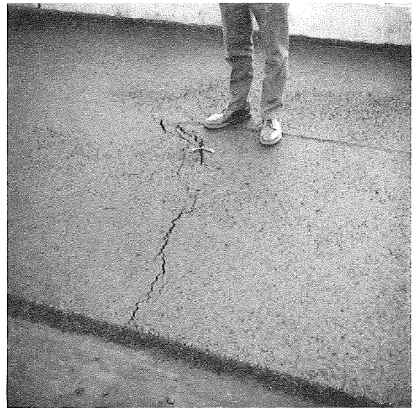
The worst of 21 cracks which occurred in the first course of pavement during the initial compaction.
