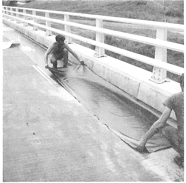
Placing 8 to 12 foot long strips on the deck so it extends up the face of the curb approximately 2 inches.
