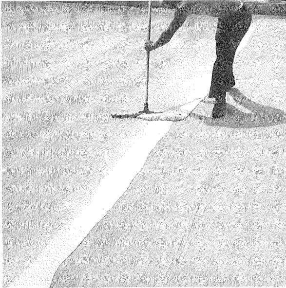
Applying first coat of epoxy cut back with 5% solvent as per manufacturer's recommendation. Application rate averaged 60 sf/gal.
