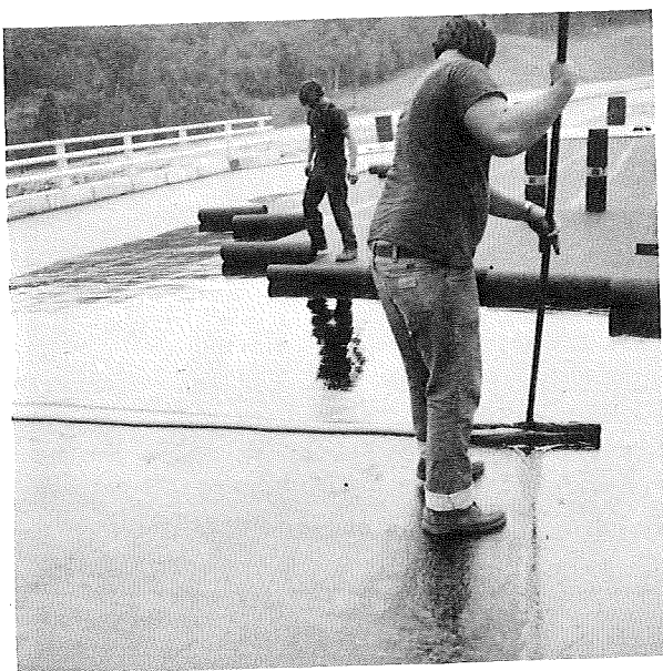
Rolling out butted 30 pound asphalt saturated roofing sheets on the freshly applied membrane.
