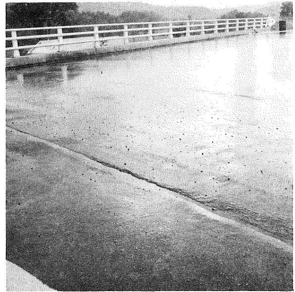
Air bubbles up to \frac{5}{8} " diameter appeared in the second coat placed over the section of prime coat which had been rained on. Many areas on the southerly end of the deck had no pinholes.
