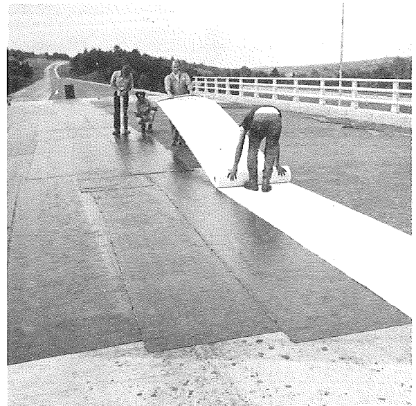
Note short strips due to difficulty in maintaining correct alignment and overlap.
