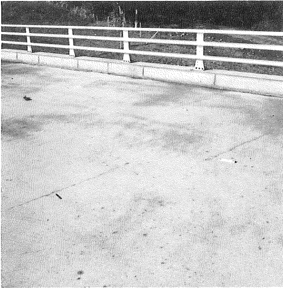
Twenty-two cracks were noted in the deck. The cracks ranged from 2.5 feet to 13 feet in length and extended through the full depth of the deck.
