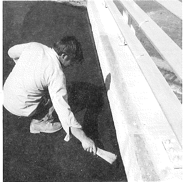
Working tar emulsion into the glass fabric extending up the curb.
