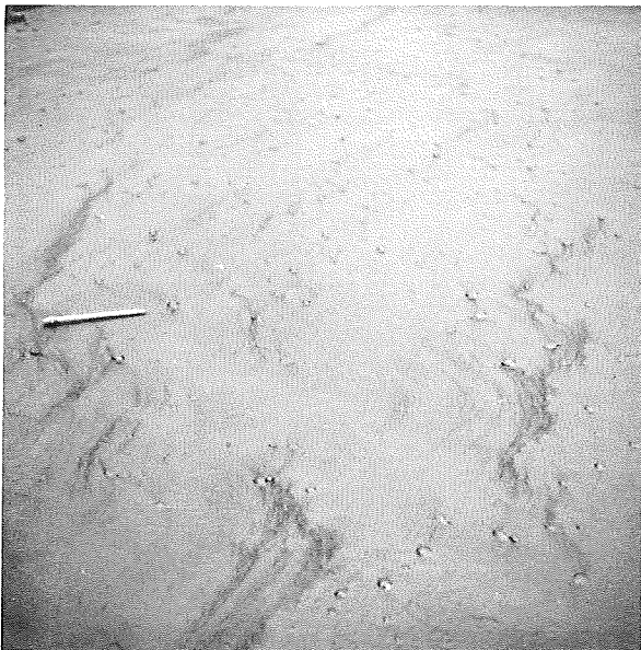
Air bubbles and ripples in the membrane left uncovered shortly after application.
