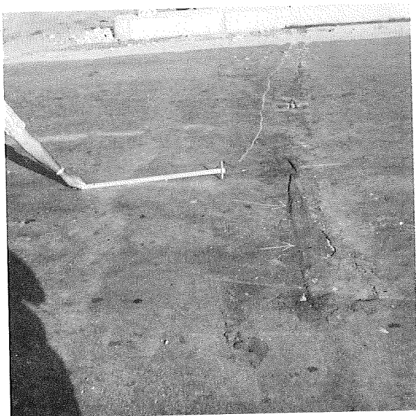
Distress adjacent to northerly approach slab includes movement of pavement and membrane which caused a bump and bleeding of the liquid membrane up through the pavement.
