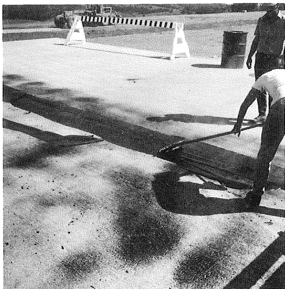
Applying liquid membrane and Elastosheet over deflection joint. Note primer application.
