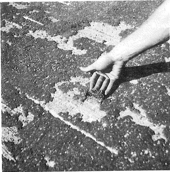
The bond between the remaining Uniroyal and the concrete allowed the membrane to be hand stripped from the deck at some locations.
