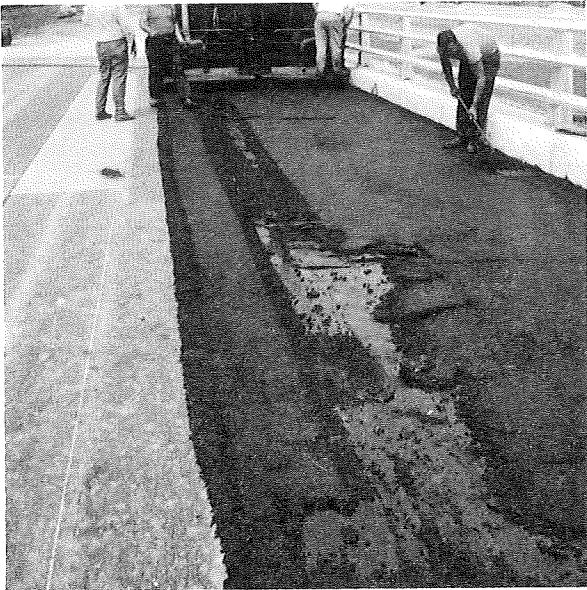
Movement of the unbonded roofing sheet caused blockage of the paver screed.
