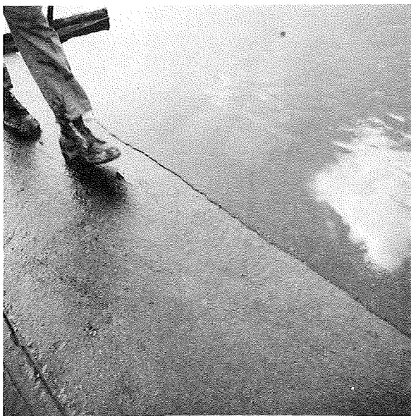
Applying second coat at an average rate of 33 sf/gal.
