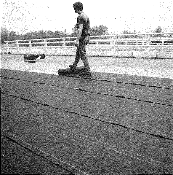
Rolling out sheets lapped in shingle fashion. Note fish mouths beginning to develop along edges.
