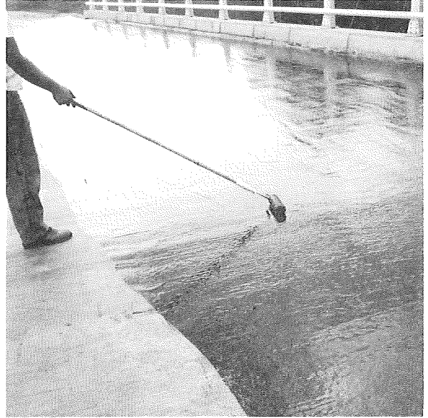
Leveling the polyurethane with a paint roller.
