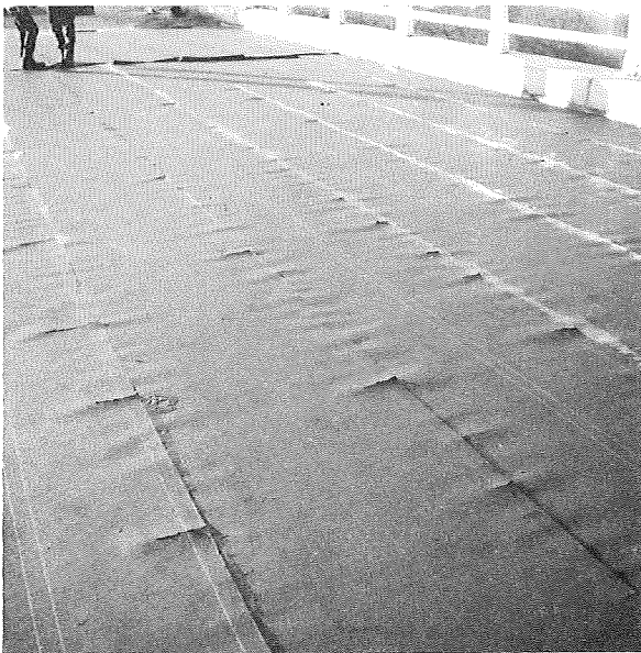
Fishmouths in the roofing sheet were cut open on the final area treated.
