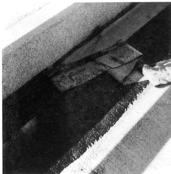
Very little bond detected between the talcum dusted Elastosheet and liquid membrane along westerly curb. Sheeting was removed.
