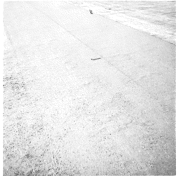
Ripples and cracks in the first 1" course of pavement were caused by the roofing sheet.
