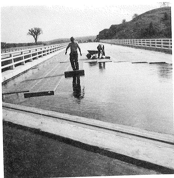
Covering the liquid polyurethane with asphalt roofing sheets.
