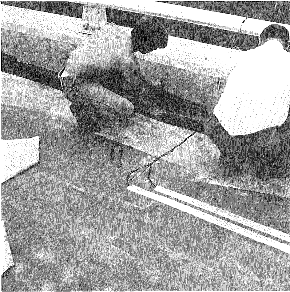
Applying 8-inch wide strips of Bituthene over bead of mastic at the curb line. Note clear primer adjacent to the curb.
