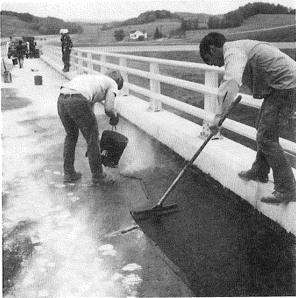
Applying second coat of liquid membrane along the curbs and over areas with holidays in the coating. Note cement dust application.
