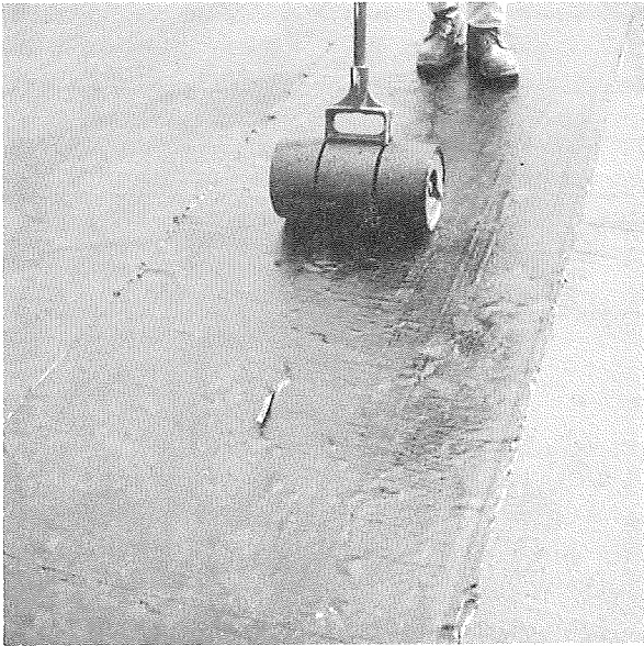
Rolling the membrane. Note entrapped air.
