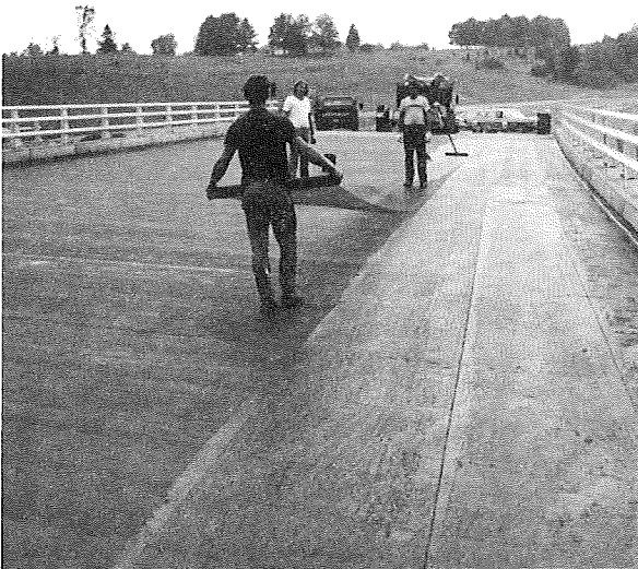
Placing longitudinal strips of glass fabric.
