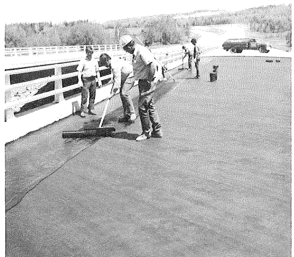
Placing longitudinal strips of glass fabric.
