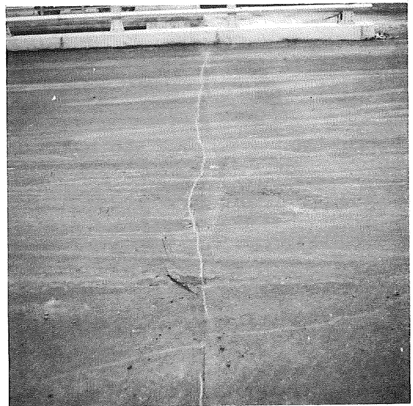
Movement of 1" thick pavement and membrane several weeks after application as indicated by keil mark on sawed pavement joint.
