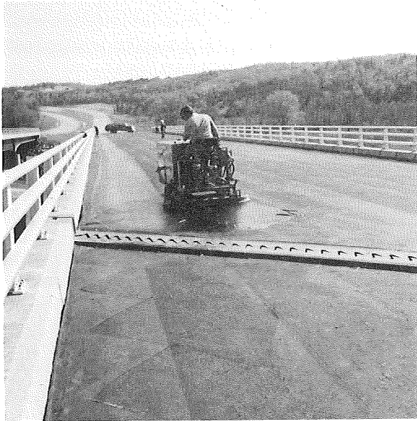
Placing final coat of tar emulsion with mechanical applicator.
