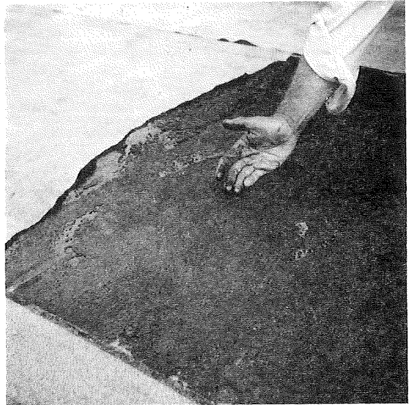
Removal of unbonded roofing sheet revealed partially cured polyurethane in some areas.
