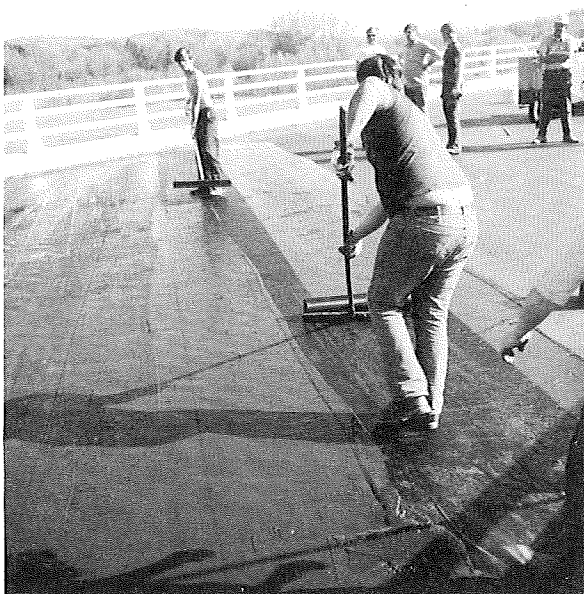
Placing transverse strips of glass fabric along the skew of the deck.
