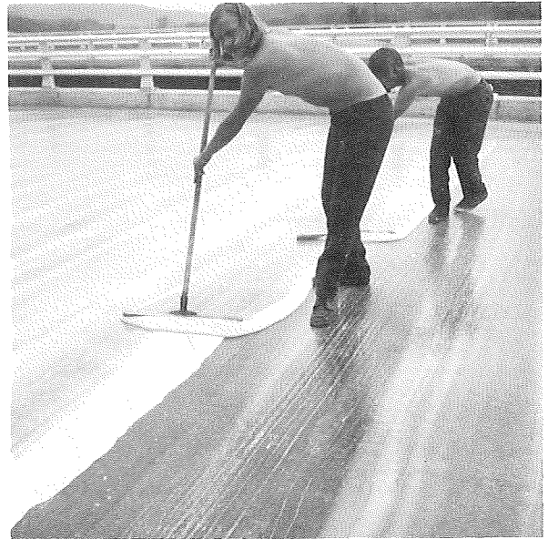
Applying second coat at an average rate of 90 sf/gal.
