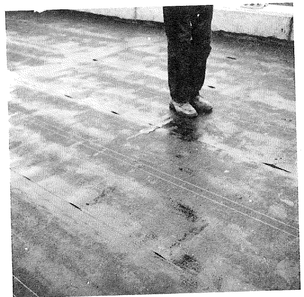
Squeezing water out from under areas of the roofing sheet which did not bond to the membrane.
