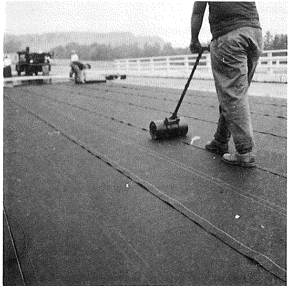
Rolling the roofing sheets in an attempt to bond the material down to the membrane.
