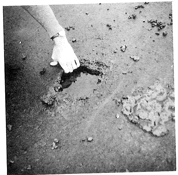
The lack of bond between pavement and epoxy is revealed by area where the hot mix stuck to the tire of a parked vehicle.
