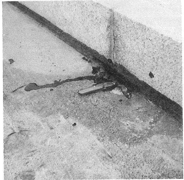
Largest of 3 areas along the westerly curb where water was able to get behind the Elastosheet before the pavement was placed.
