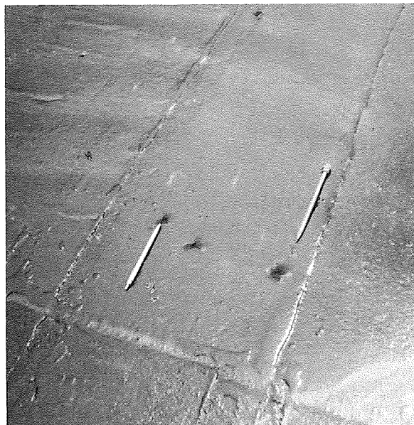
Bubbles noted in liquid membrane shortly after application. All revealed concrete when broken open.
