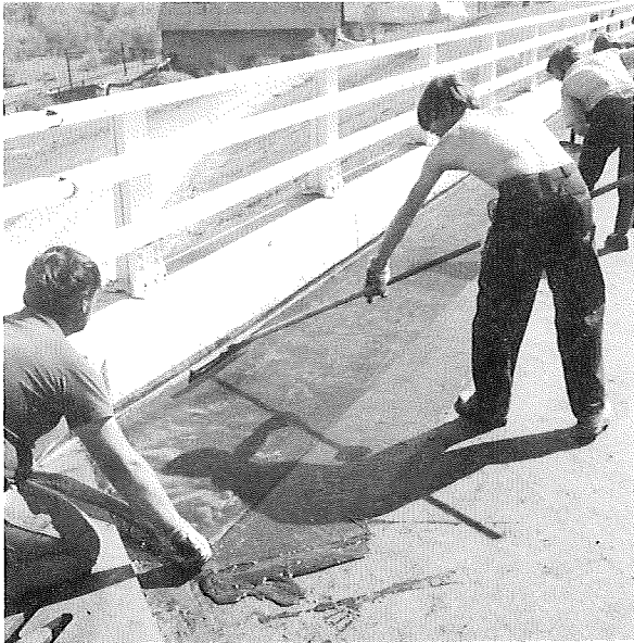
Placing the second coat of glass fabric along the curb.
