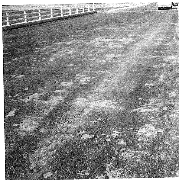
Removal of the distorted pavement with a grader resulted in exposed areas of concrete where the Uniroyal stuck to the bituminous mix rather than the concrete deck.
