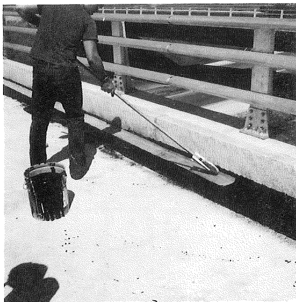
Forcing the Elastosheet into the liquid membrane at the joint between deck and curb.
