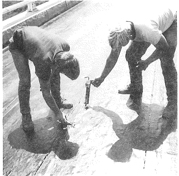
Puncturing large air bubbles and sealing the holes and overlaps with mastic.
