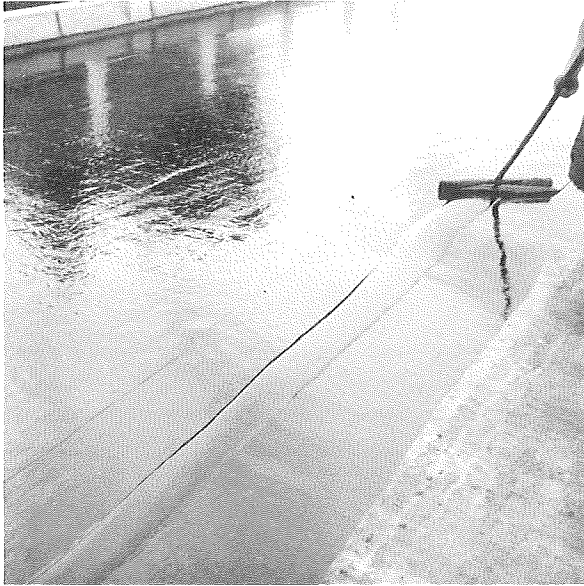
Applying the polyurethane with a squeegee. Note asphalt droppings and prime coat on concrete.
