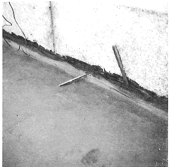
Curb area not properly sealed.
