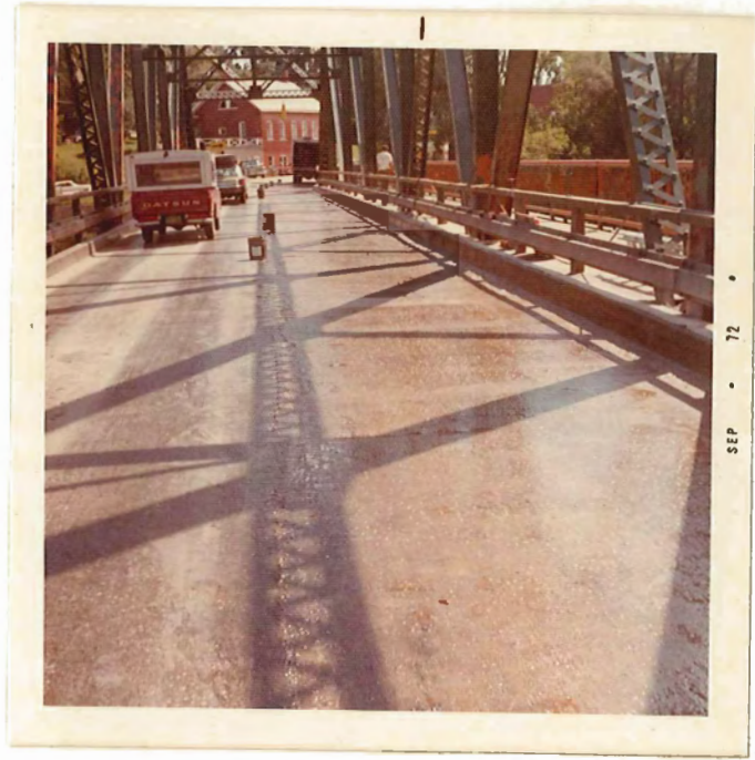
First coat complete on southbound lane
